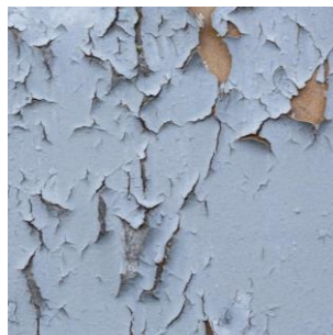
图 9: 漆面剥落 [11]
