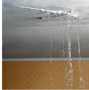
Figure 7: Roof leakage [9]
