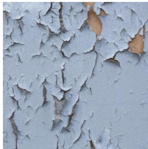
Figure 9: Peeling paint [11]
