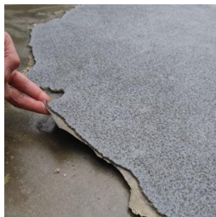
Figure 2: Waterproofing Failure [4]
