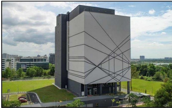
Figure 2: AIMS Data Centre in Putrajaya [10]
