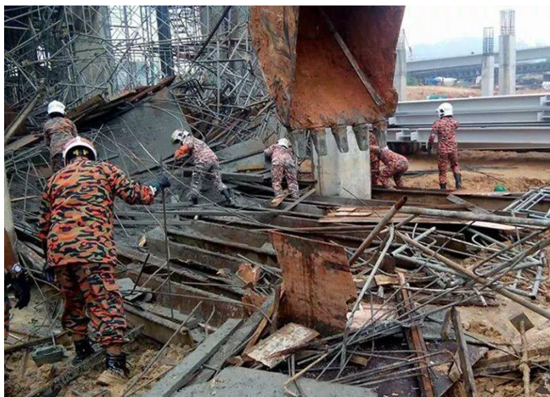
Figure 7: Failure of Temporary Works (Falsework) [13]
