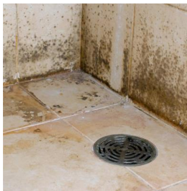
Figure 2: Bathroom mold [8]
