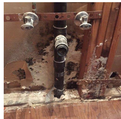
Figure 3: Mold growth due to leaking pipe [9]
