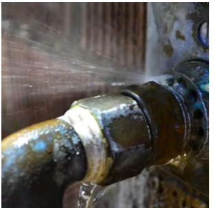
Rajah 8: Paip lama bocor [10]
